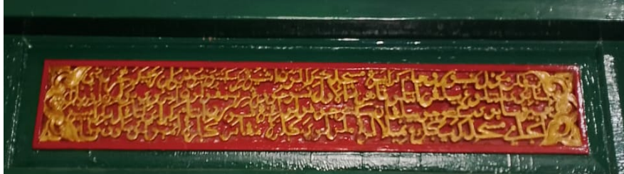
Figure 3. North Gate of the Old Al-Hilal Katangka Mosque
